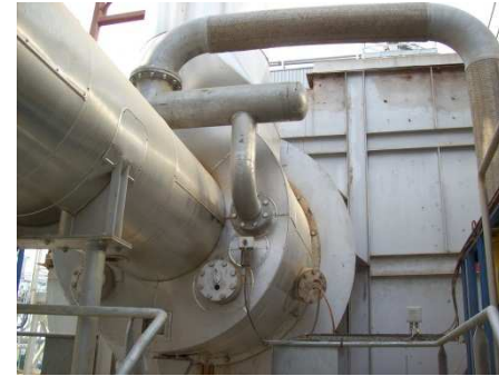
Natural gas burner
